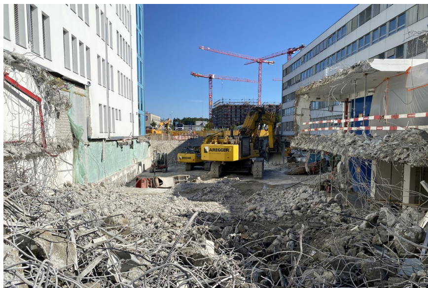
Baustelle Zwihatt, September 2022 / © GMS Partner AG, Zürich
