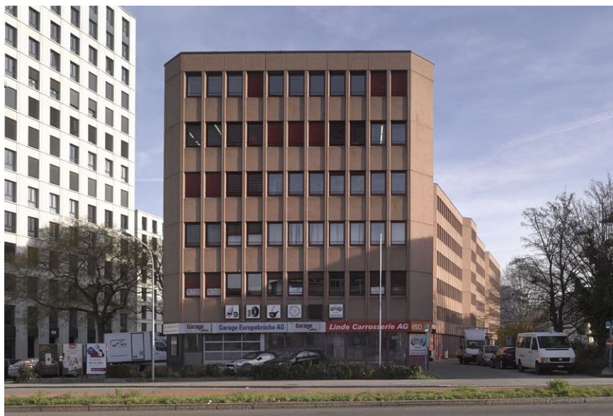
Westfassade Albulastrasse 57 in Zürich-Altstetten / © Pensimo
